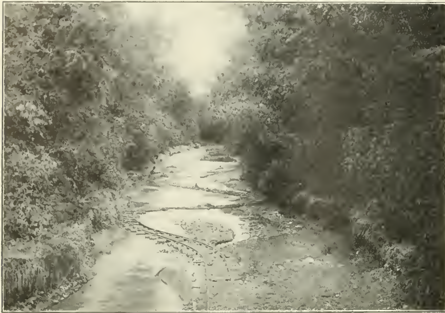
TRACK TO GRAVEL PIT, PHILIPPINE RAILWAY, CEBU, P. I.
